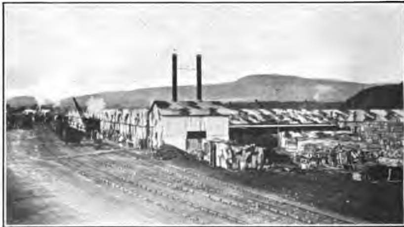
ASSEMBLY SHOPS AND READY ISSUE STORE AT BASE 18.
