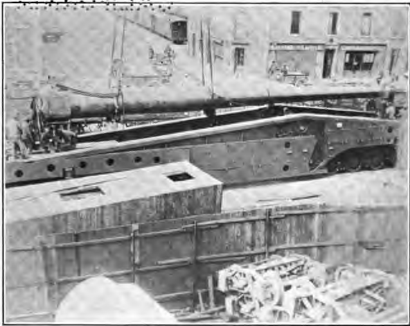
PLACING 14-INCH 50-CALIBER GUN ON GIRDER FOR TRANSPORTATION TO THE SHOPS.
