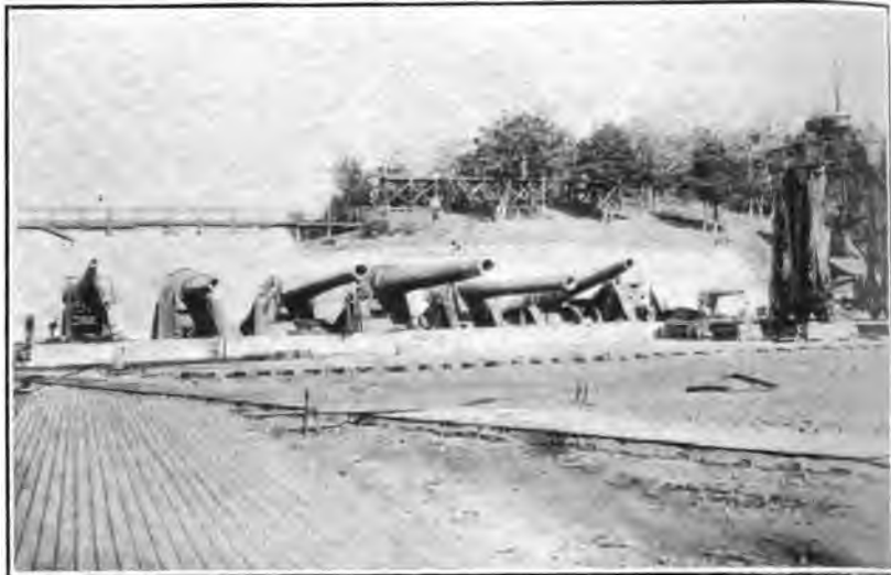
RANGING BATTERY IN THE VALLEY AT PROVING GROUND, INDIAN HEAD, SHOWING GUNS OF LARGE CALIBER, OBSERVATION PLATFORMS, AND, AT THE RIGHT, A GANTRY USED FOR TRANSPORTING GUNS.
