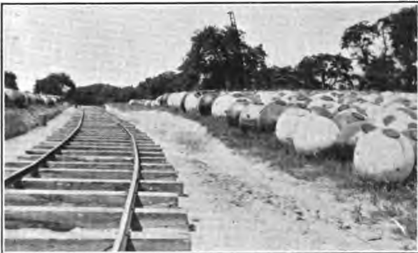
MINES STORED IN THE OPEN AT NAVAL MINE DEPOT, YORKTOWN, VA., AWAITING COMPLETION OF STOREHOUSES.
