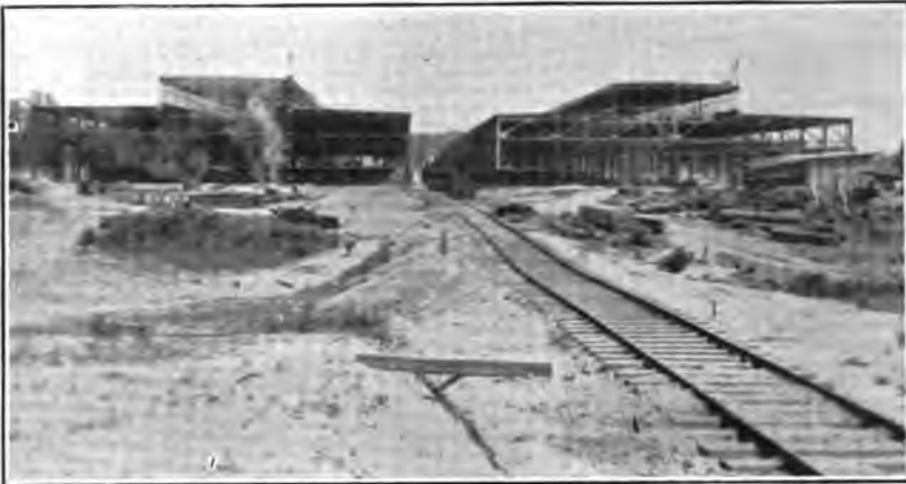
MINE STORAGE BUILDINGS UNDER CONSTRUCTION AT NAVAL MINE DEPOT, YORKTOWN, VA.
