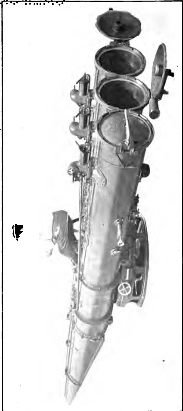
ABOVE WATER, 21-INCH TRIPLE_TORPEDO TUBE, FOR USE ON DESTROYERS.
