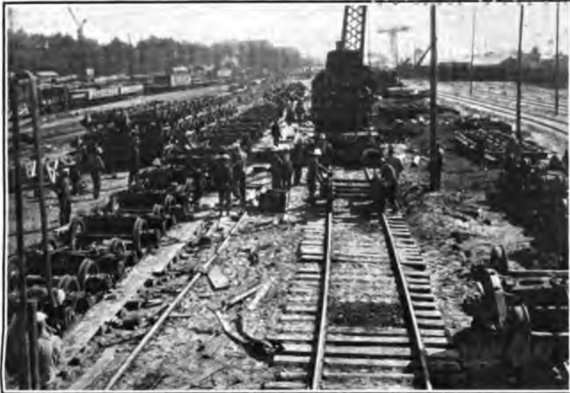
ASSEMBLING TRUCKS FOR CARS OF THE U. S. NAVAL RAILWAY BATTERIES, ST. NAZAIRE, FRANCE.
