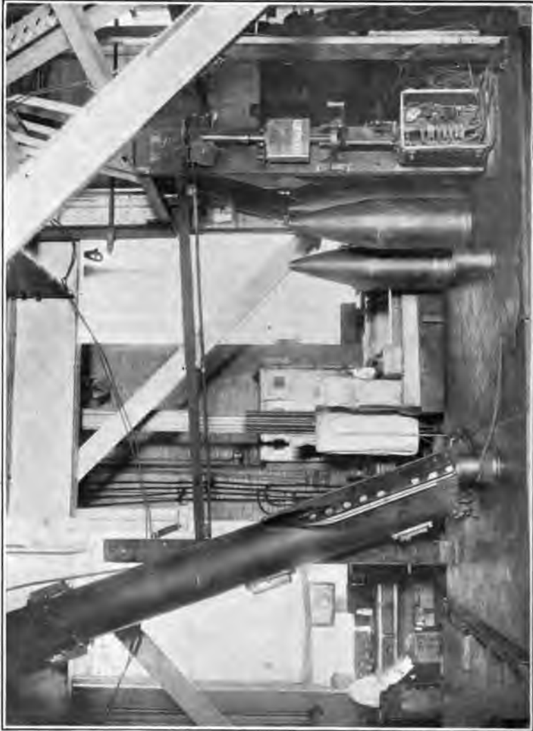
BOTTOM OF 14-INCH SHELL HOIST, SHOWING PROJECTILE, TUBE-HOIST CONTROL MECHANISM, CAPSTANS FOR PARBUCKLING, AND MOTOR CONTROL.
