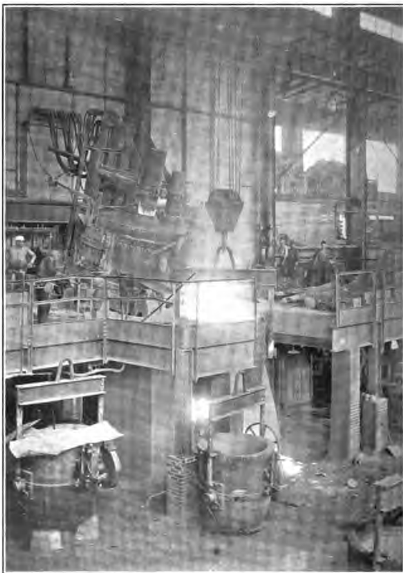
ELECTRIC FURNACE, NAVAL ORDNANCE PLANT, SOUTH CHARLESTON, W. VA.
