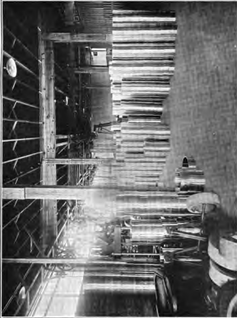
14-INCH COPPER ROTATING BANDS READY FOR ASSEMBLY ON PROJECTILES.
