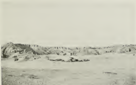
DUG-OUTS IN THE FRONT LINE, SHEIKH ABBAS.
