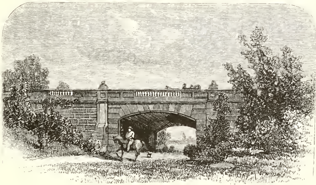
BRIDGE OVER THE BRIDLE PATH NEAR ARSENAL.
