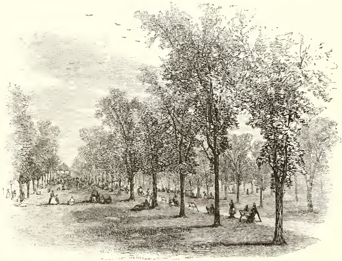
THE MALL, LOOKING UP.
