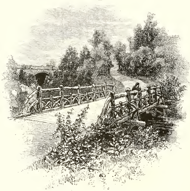
RUSTIC BRIDGE, NEAR BALCONY BRIDGE, LOOKING EAST.
