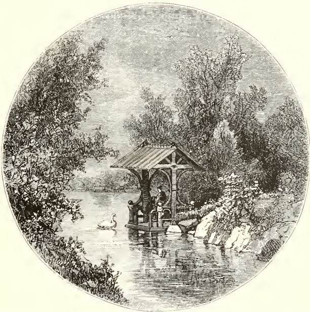
BOAT HOUSE NEAR OAK BRIDGE.
