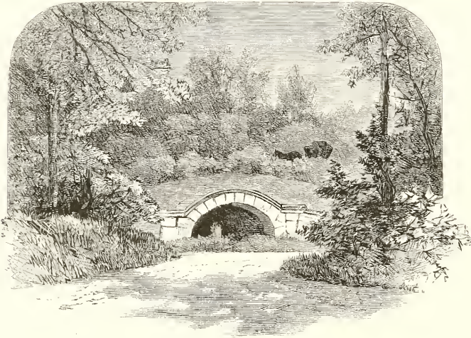
ARCH OVER FOOT-PATH NEAR RAVINE.
