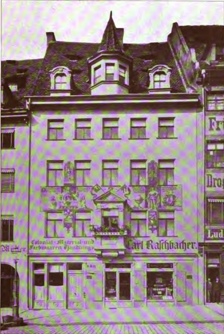
THE "BEHAIM" HOUSE AT NÜRNBERG.
