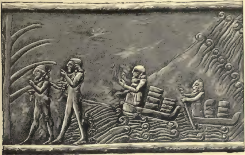
TRANSPORT OF BUILDING MATERIALS BY WATER. 2
